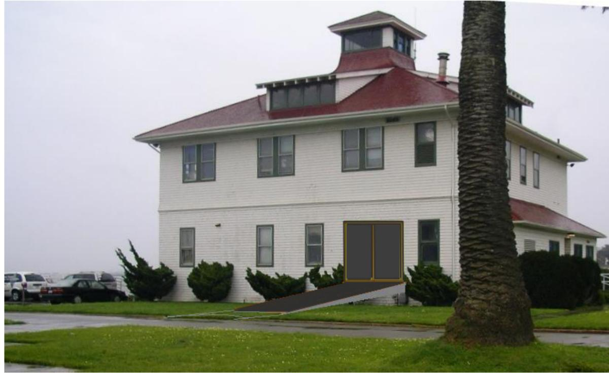
[7]: *Proposed Boathouse Ramp (Building 1903): This ramp is an artist's rendering of a recreated ramp to the boathouse, in its pre-existing location that provides access to the re-constructed boathouse doorways. Colors of non-skid ramp surface, doors and trim to be submitted to GGNRA for review. (Photo and illustration by NPS staff, 2007.)*
