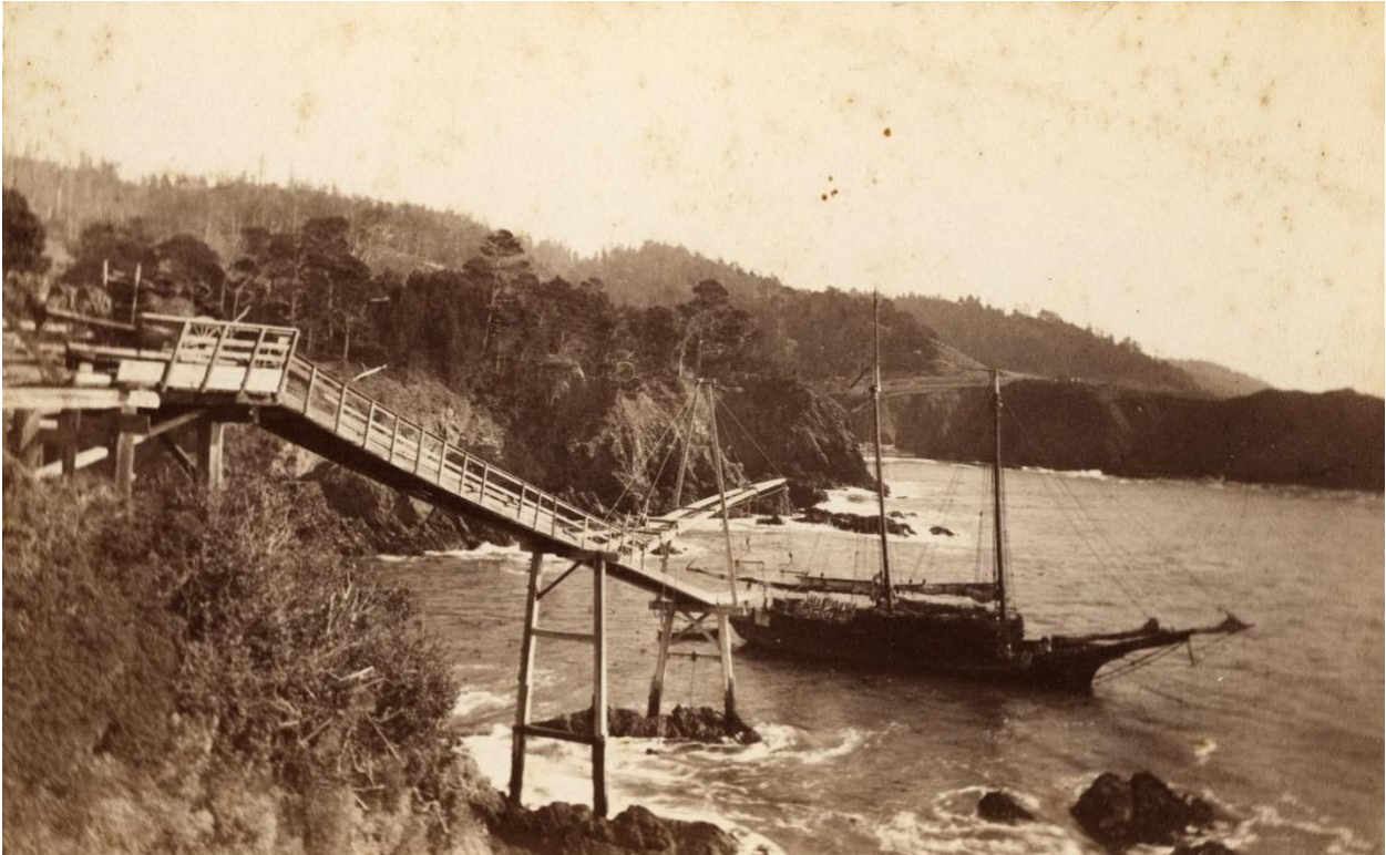
Figure 7. Trough chutes at Stewart's Point Landing and unknown schooner loading tanbark. Photo: San Francisco Maritime National Historical Park SAFR 21374.
